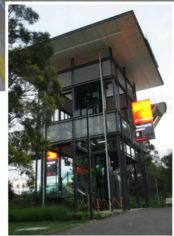
Pictured: Yerrongpilly, Qld, Railway Station pedestrian flyover utilising the MFAPC128
